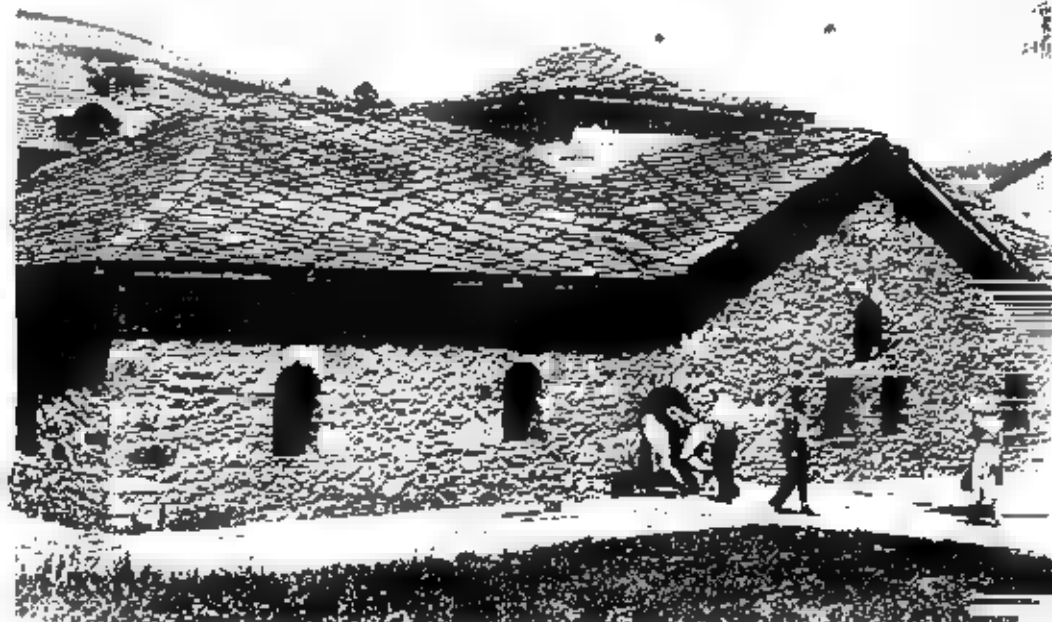
1a. The Church ■ Barak where a large number of people died during the April Rising. Architecturally the church is of interest because it belongs to the period when the Turks placed severe restrictions ■ the height and style of Christian buildings.
